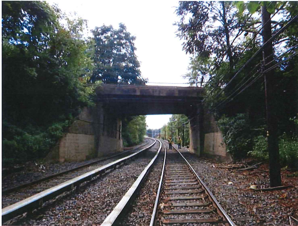
Church Road Bridge, Left Elevation
