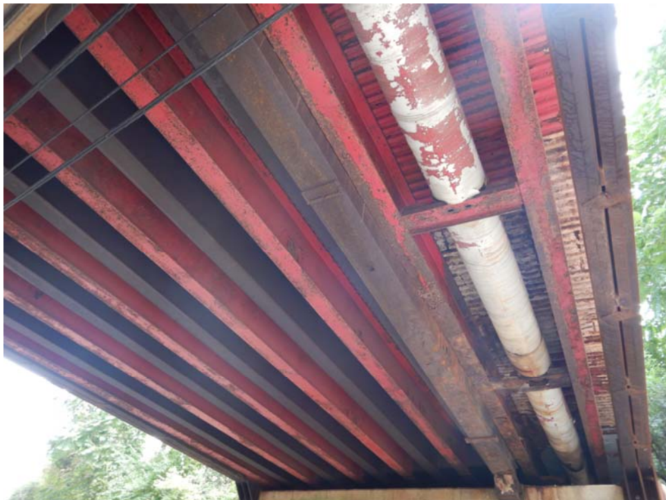
Superstructure, looking ahead.
