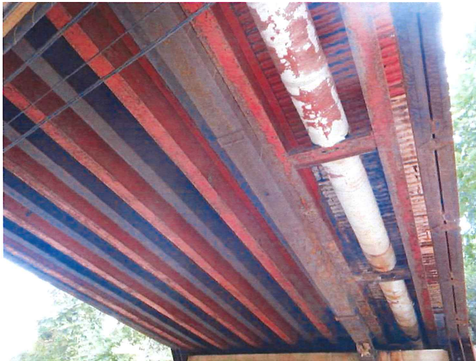
Superstructure, looking ahead.
