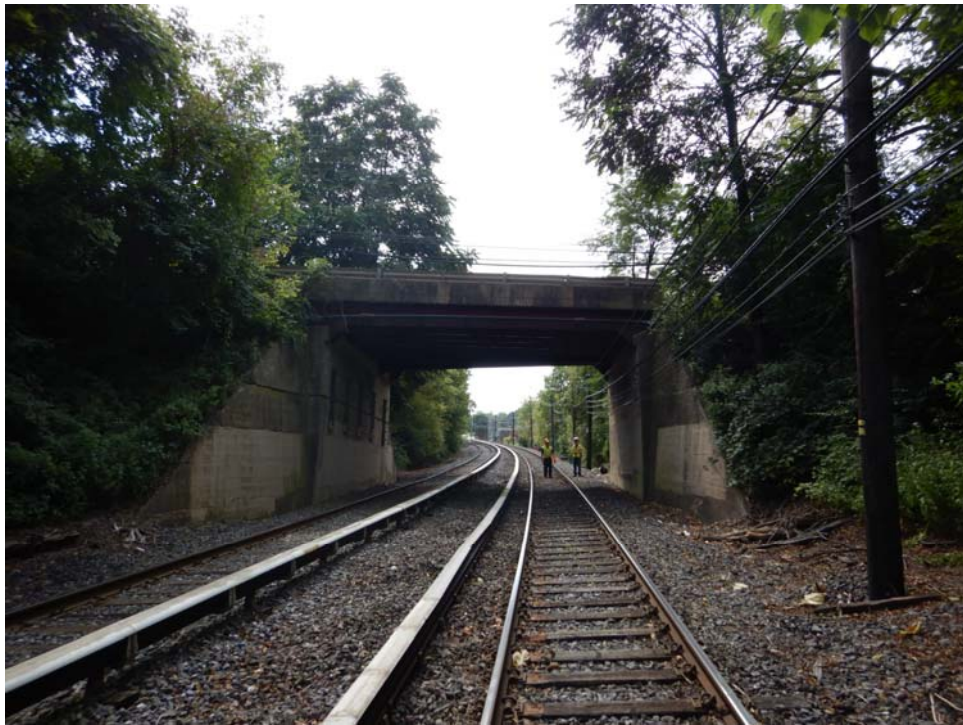
Church Road Bridge, Left Elevation
