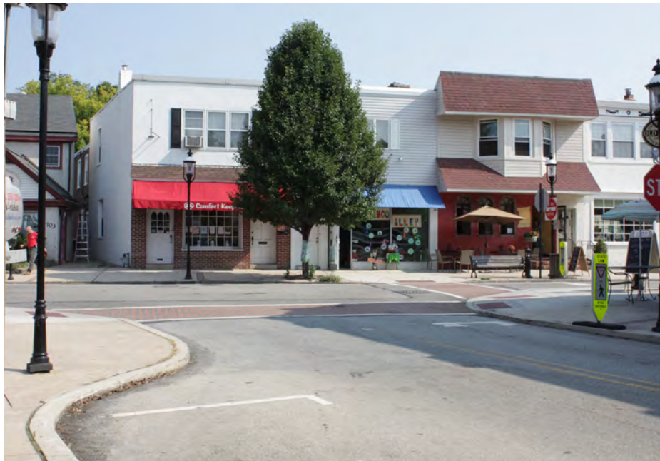
Traffic Calming Curb Bumpout in Bridgeport Borough
