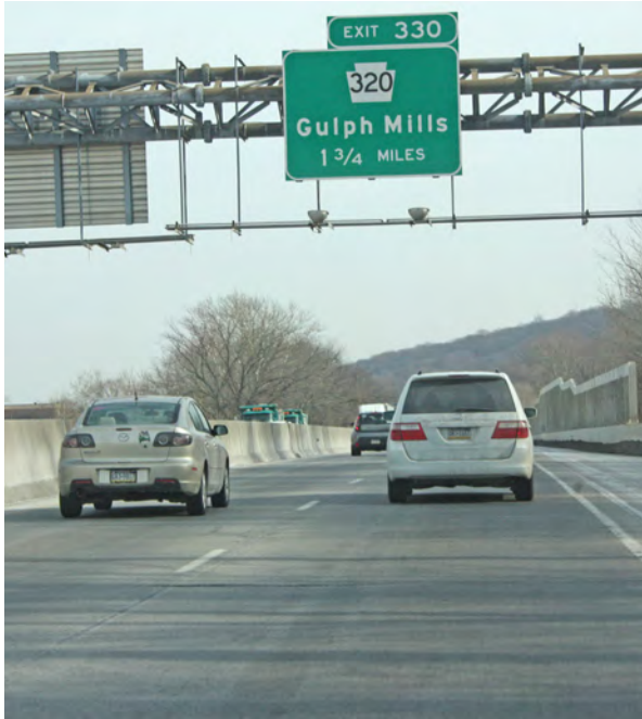
Schuylkill Expressway at Gulph Mills
