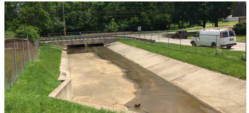
Concrete Basin in Swedeland
