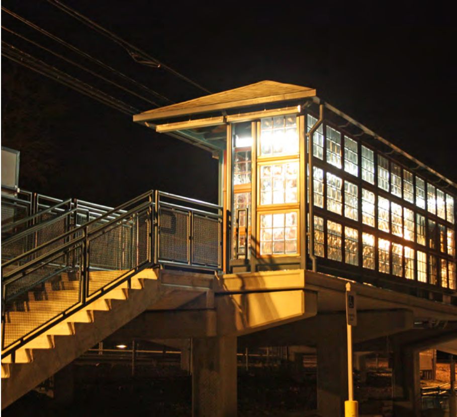
Gulph Mills NHSL Station at Night
