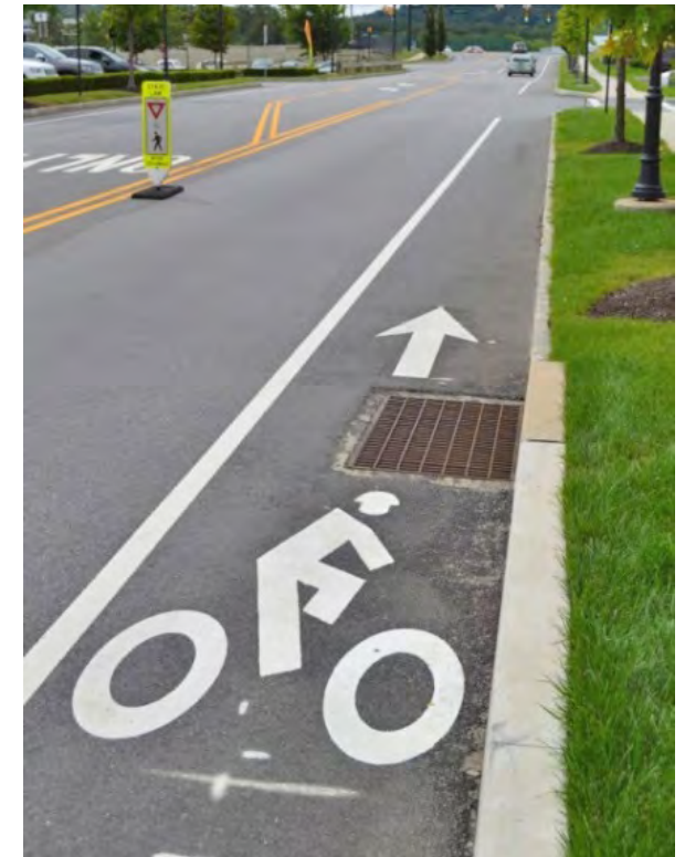
Bike Lanes at Village at Valley Forge
