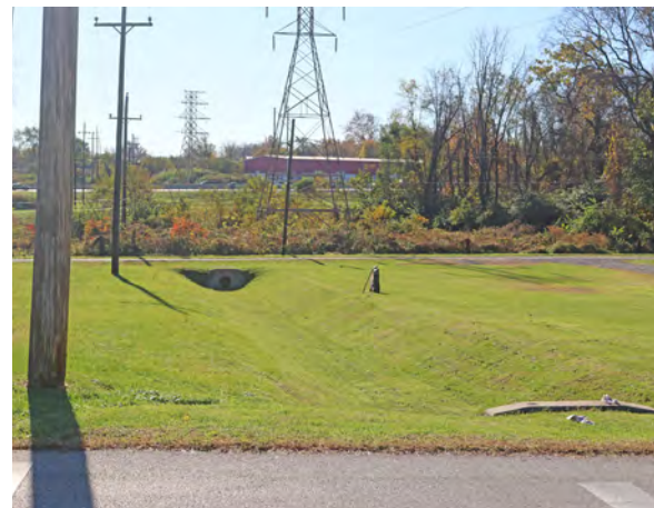
Stormwater Drainage on Coates Lane
