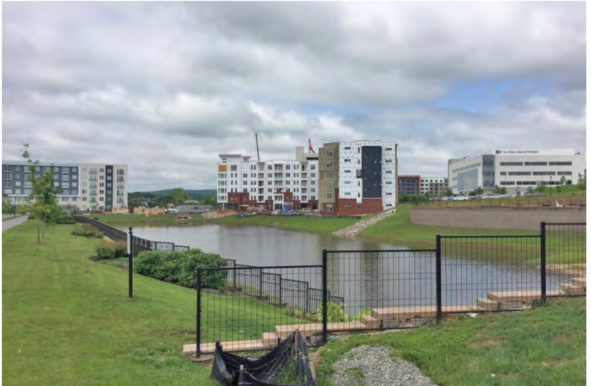
Construction at Village of Valley Forge
