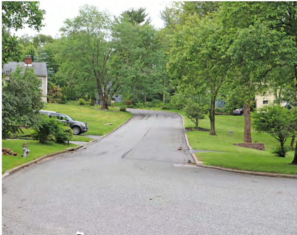
Hansen Road Street Conditions and Lack of Sidewalk at Sweetbriar Park
