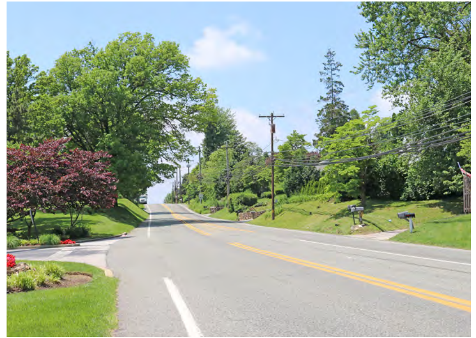
Missing Sidewalks along S. Gulph Road
