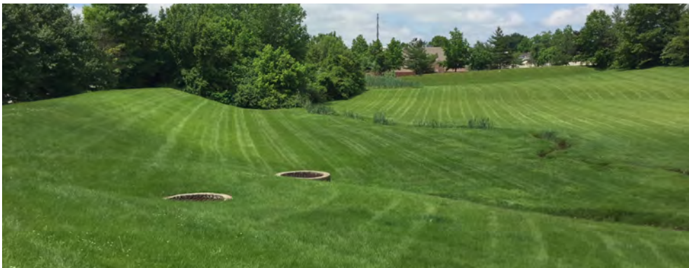
Stormwater Basin in Swedeland Area
