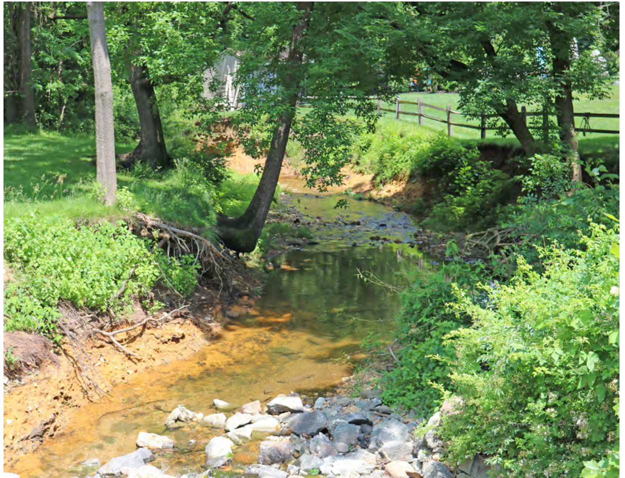
Example of Stream Erosion
